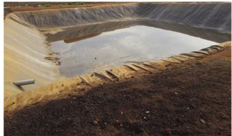
Treated water storage
